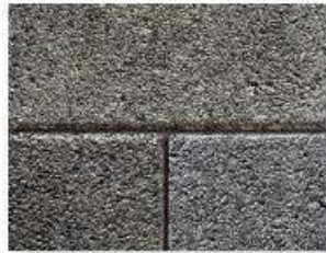
Exposed Aggregate Finish
