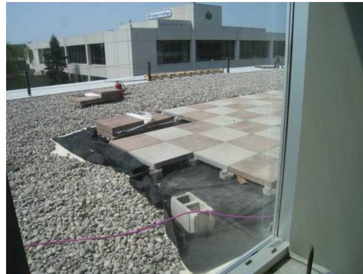
College of DuPage Culinary and Hospitality Center, Glen Ellyn, IL (2011) The paver on the roof deck was matched with the paver used on-grade.
