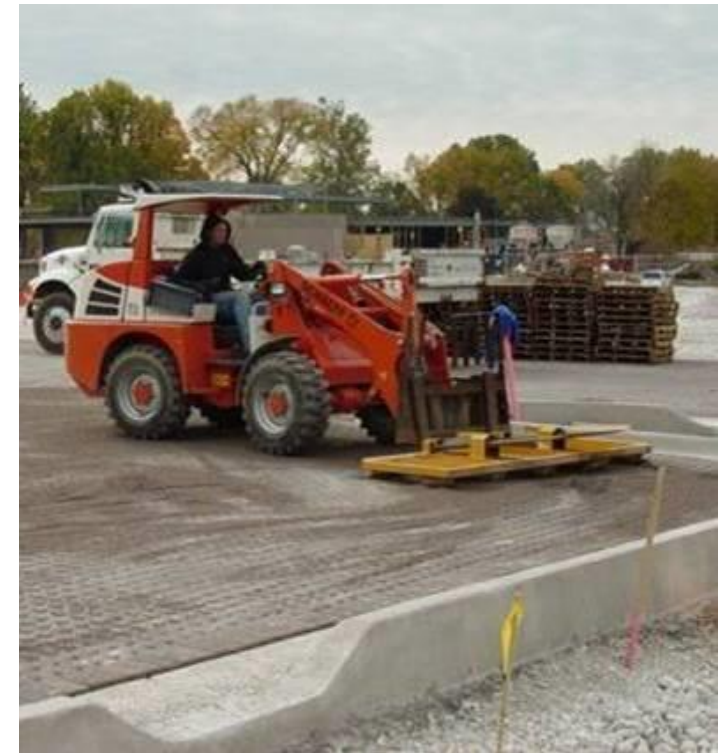
Mechanical joint filler.
