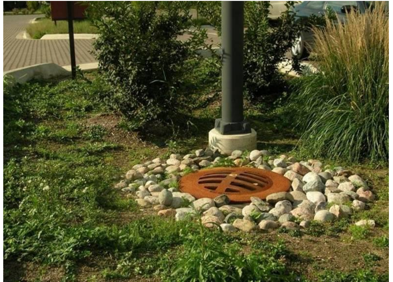
A raised inlet (to force infiltration) and vegetated swale work in concert with PICP.
